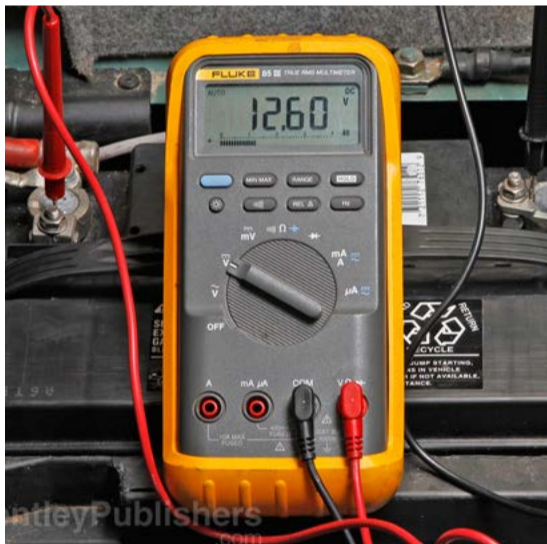
Battery voltage should be about 12.6 V DC with the engine off. (Chapter 2, "Battery")
